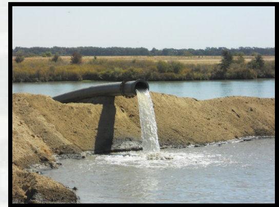
Hydraulic Dredging and upland placement along the Sacramento Deep Water Ship Channel, CA
