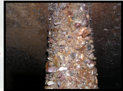
Deteriorating concrete in Tappan Lake tunnel liner – exposed aggregate
