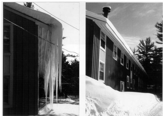
**Figure 1** Two identically constructed roofs photographed at the same time. The one on the right, with no icings, was unheated.
