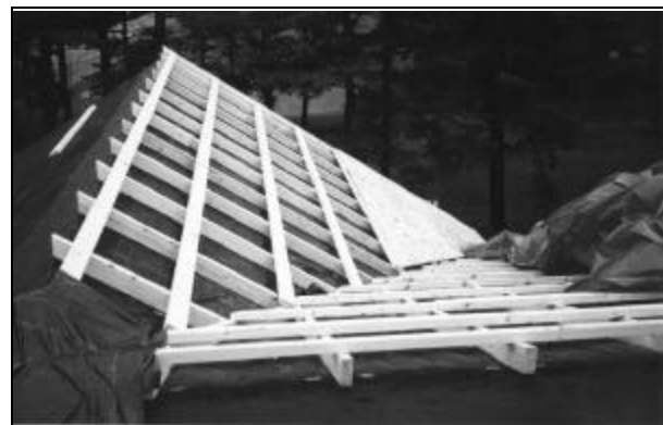
Figure 14. Cross-purlins allow ventilation of this valley.
