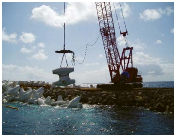
Figure 18. Core-locs and Core-loc placement on the jetty at Kaunalapau Harbor, Lanai, HI in 2007.
