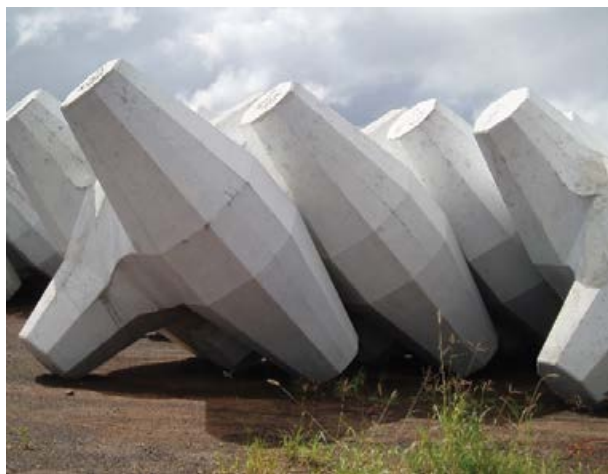
Figure 18. Core-locs and Core-loc placement on the jetty at Kaunalapau Harbor, Lanai, HI in 2007.
