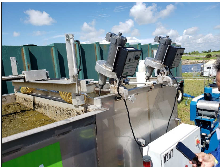
Figure A-13. Conditioning compartment of the HABITATS where coagulants and flocculants are added and mixed into the algae contaminated solution.
