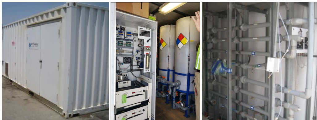
Figure 2-11. Containerized ozone advanced oxidation system from HiPOx, Inc. The system is capable of treating with ozone or ozone plus hydrogen peroxide.
